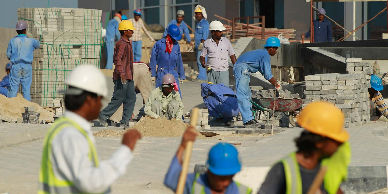
Foreign workers lay an entrance road at the construction site of a new hotel in the new City Center and West Bay district on October 24, 2010 in Doha, Qatar. (Photo by Sean Gallup/Getty Images). © 2010 Getty Images
